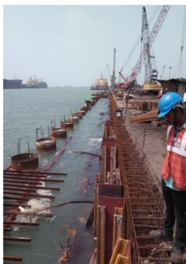
EXISTING BERTHS BEING STRENGTHENED, WIDENED & DEEPEMED
