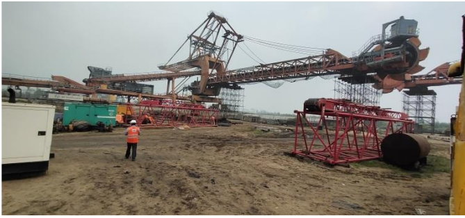
STACKER/RECLAIMER UNDER INSTALLATION
